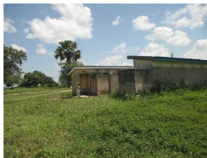
One of the school toilets in need of repair.
